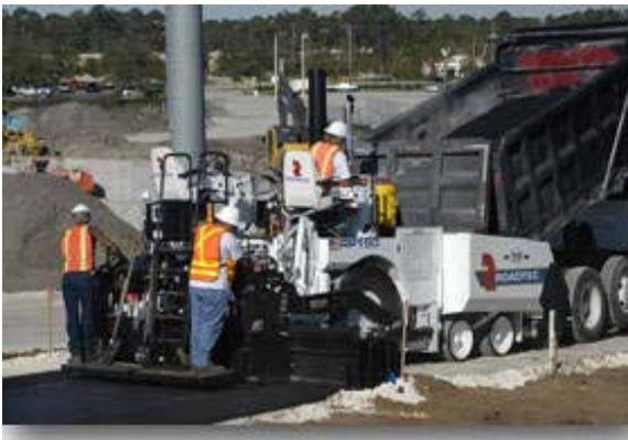
***Sample of an asphalt paving machine***
